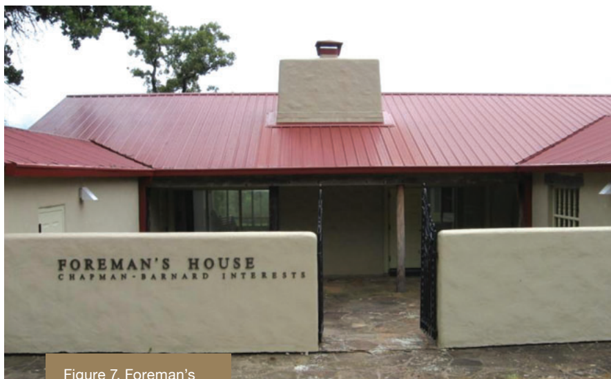
Figure 7. Foreman's House at the TGPP. Photo / Matt Allen
